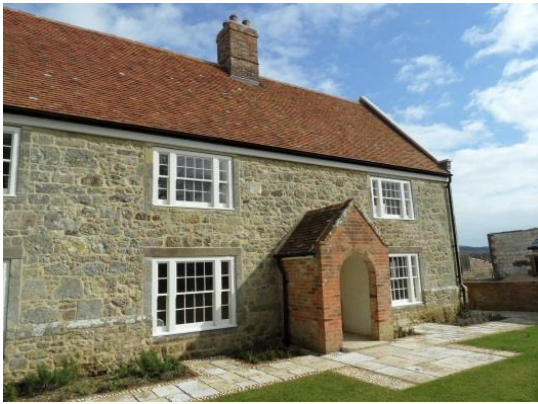
Little Budbridge Farm House
